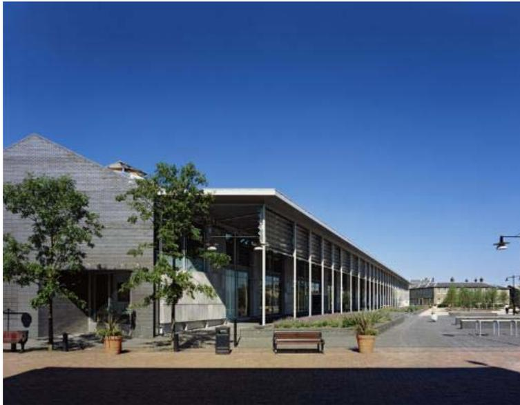
The building is designed to be naturally ventilated, with exposed mass concrete slabs, motorised openable windows and those roof snouts that draw air through the building. An array of photovoltaic panels on the roof provides some 30% of the annual electricity requirement. All this provides the National Trust with low energy consumption and low running costs.
