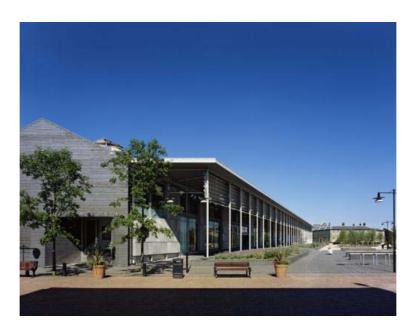
The building is designed to be naturally ventilated, with exposed mass concrete slabs, motorised openable windows and those roof snouts that draw air through the building. An array of photovoltaic panels on the roof provides some 30% of the annual electricity requirement. All this provides the National Trust with low energy consumption and low running costs.
